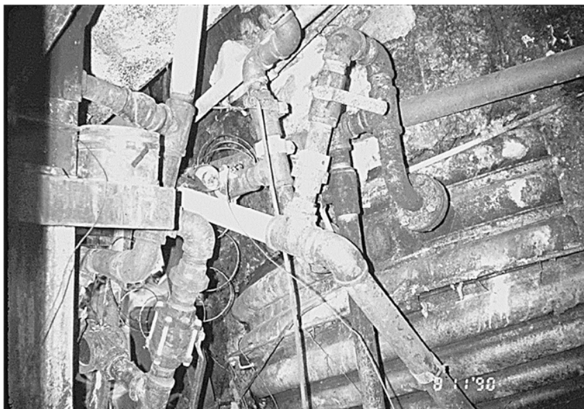
Figure 8.3 As-found Position of Valves—Example Photo
